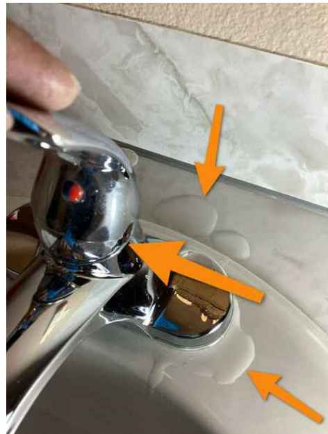
Bathroom - Lower Level
