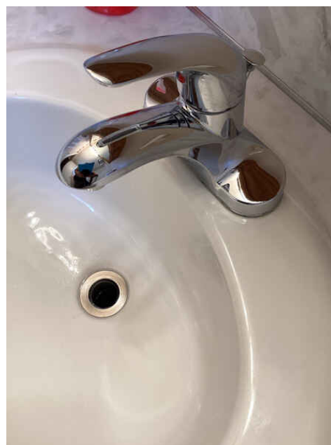
Bathroom - Lower Level
