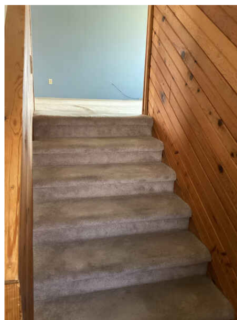
Upper Level Stairs
