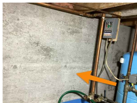
East - Under Stairs Foundation Wall
